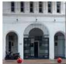
Pillars in front of the veranda to prevent strong sunlight into the building.
